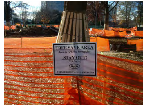
Tree protection during construction.
